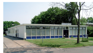
Fig. 1: Former building of REGULATEURS EUROPA
